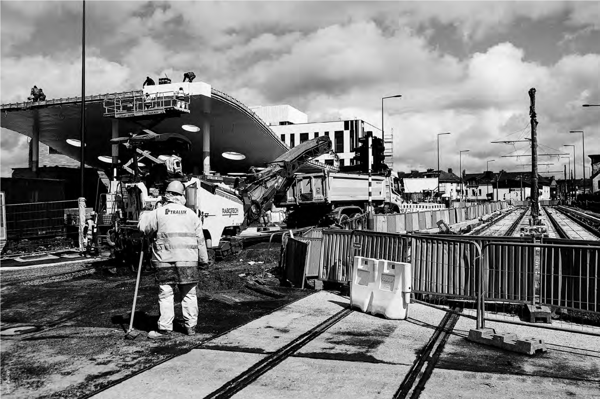
Tram-Baustelle in Howald
