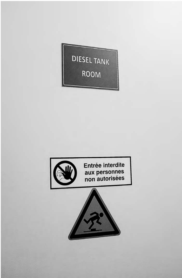
The increasing digitalisation across all business sectors will massively drive demand for low-carbon electricity – Data center in Luxembourg-City
